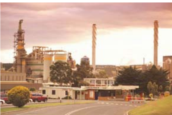
Entrance to the Maryvale mill
